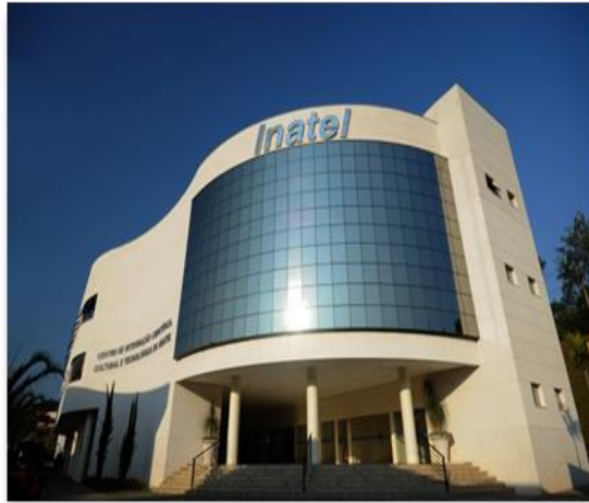
Building V Frontage
